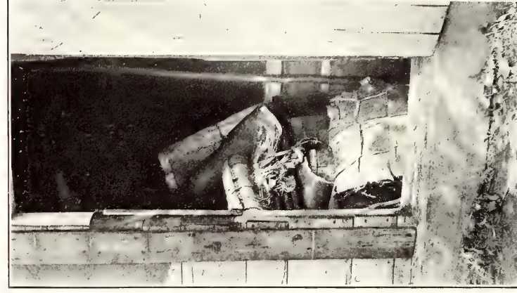
c, STORAGE SHED (OPEN)
